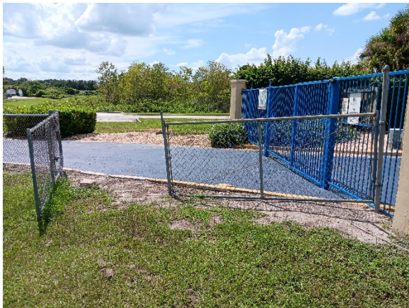
Access gate to easement
