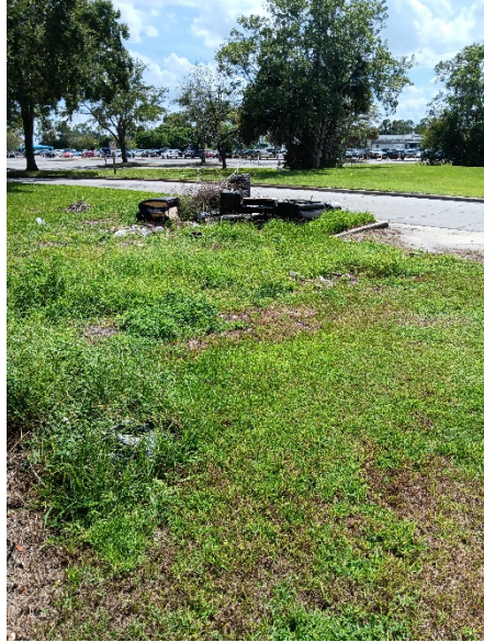
Close-up of material staging area Sea World Dr
