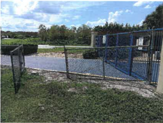
Access gate to easement
